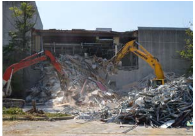
Owings Mills Mall, which closed in January, is expected to be completely demolished by the end of the year.
