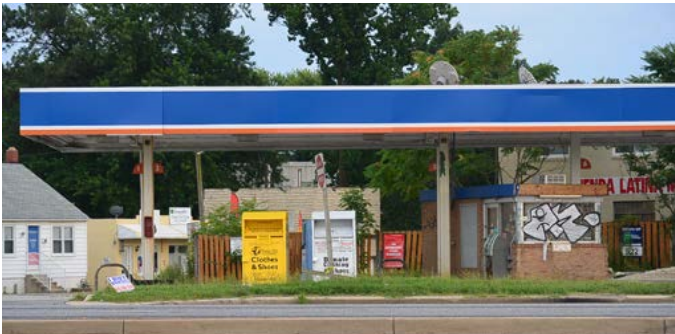
Clockwise, from top: While the Security Boulevard area in Woodlawn has the federal Centers for Medicare and Medicaid Services and Social Security Administration, it also has several vacant buildings: a long-closed McDonalds that was burned in August, the former Ben-nigan's and IHOP restaurants at Security Square Mall, Wendy's at Whitehead Road, and an office building across from Social Security Administration. To the left is the shuttered Gulf gas station on Baltimore National Pike at Winters Lane in Catonsville.
